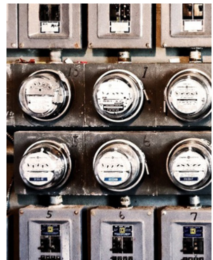
Figure 22: Submetering tenants for heat and electricity will allow Teatown to determine if there are any energy inefficiencies in those spaces. (Source: Aquicore )
