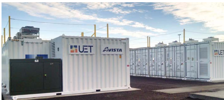
Figure 29. The State of Washington's Avista Utilities energy storage project involves a 1 MW, 3.2 MWh large-scale flow battery system
