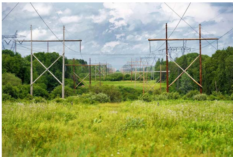
Figure 44. Wooden H-frames like these pictured need to be updated to steel monopoles to improve aging transmission infrastructure in New York
