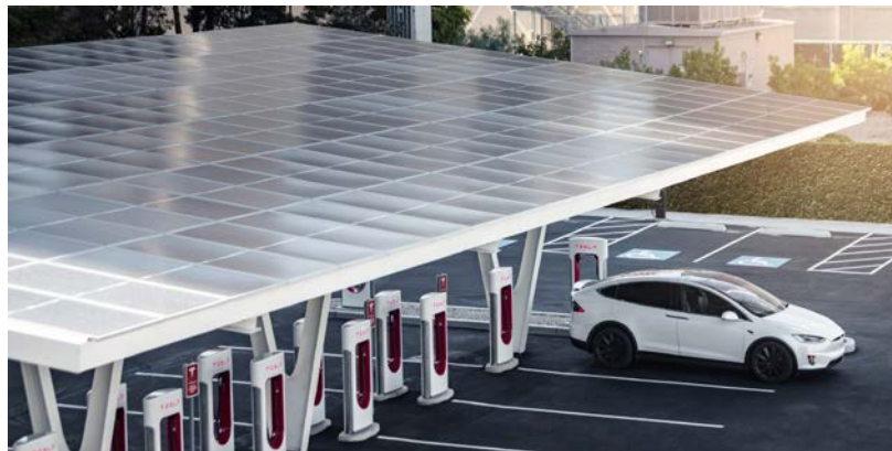
Figure 39. A Photovoltaic Solar and Battery Energy Storage System Electrical Vehicle Station
