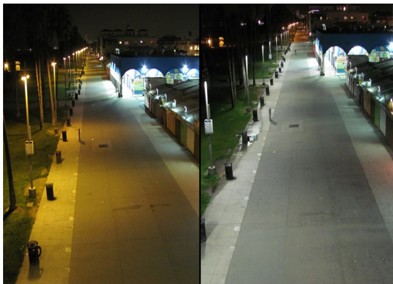
Image LT2: Los Angeles Street Lights Before and After LED Replacement 229
