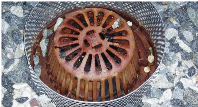
PHOTO 9: BLUE ROOF FLOW RESTRICTOR. PHOTO CREDIT: PLANYC
