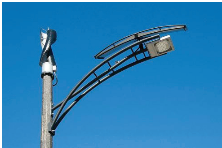
Figure 40 - Wind and Solar-Powered Lamp Posts 17
