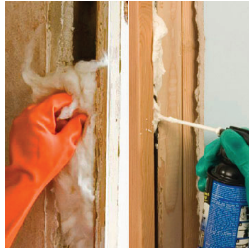
Figure 22 - Insulating a Window Cavity
