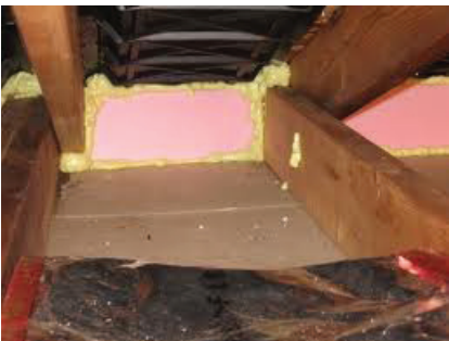
Figure 50 - Attic Sealing of Gap in Eaves
