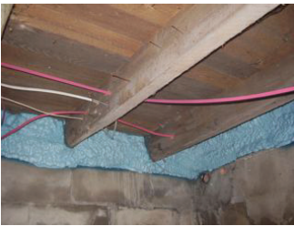
Figure 49 - Basement Sill – Spray Foam
