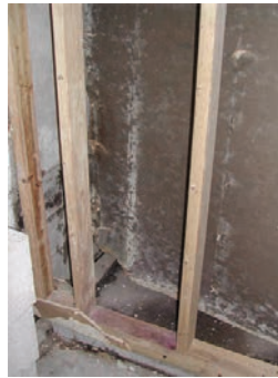
Figure 46 - Mold in a Wall Cavity
