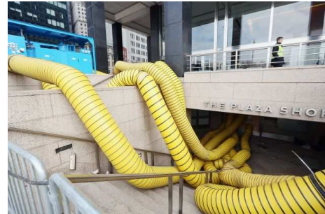
Figure 4-2: Air tubes dry out lower levels of commercial building following Hurricane Sandy (Photo Source: Stamford Advocate)
