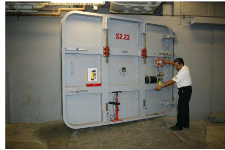
Figure 5-1: Submarine type doors installed at Texas Medical Center after severe flooding from Tropical Storm Allison (Photo Source: Times Free Press)
