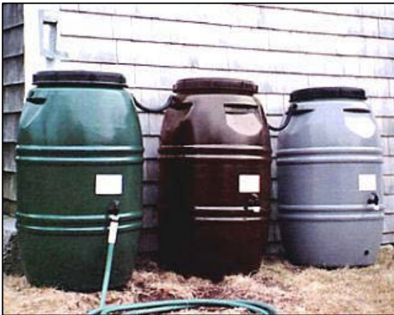
Figure 15. Three 60-gallon barrels linked in series (Buffalo Niagara Riverkeeper).
