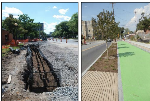
Figures 12 and 13. Silva Cell installation and tree installation before and after (Onondaga County, New York).
