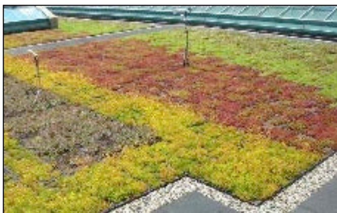
Figure 14. Con Edison green roof modular system after one year, with two sensors that measure radiant energy absorbed by the roof, ambient air temperature, relative humidity and wind speed and direction (Gaffin, Rosenzweig and Khanbilvardi).
