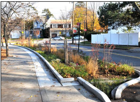
Figure 10. This bioswale, located in Jamaica Bay, Queens, helps to control the flow of stormwater runoff and decrease localized flooding (Ulam).
